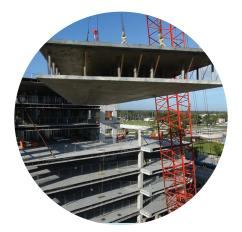
The DualDeck® Building System revolutionizes durable concrete material and cuts construction time down significantly by allowing sub-trades to work on the project in concurrent phases.
